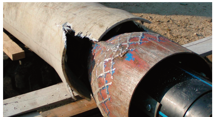
Demonstration of the bursting head, penetrating the existing pipe
