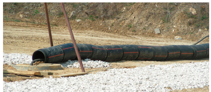
Feeding of the bursting equipment with HDPE pipe sections
